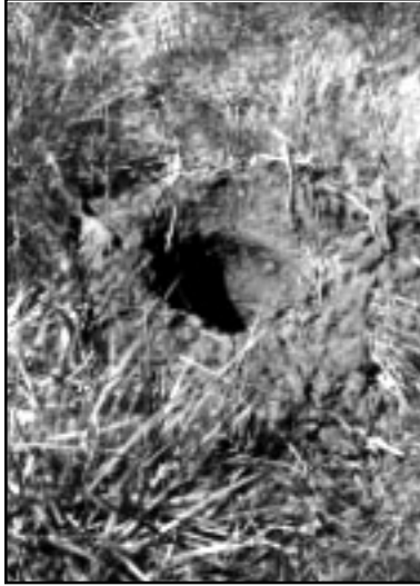
BURY THE BURROWS. Fill animal burrows quickly to prevent destabilization.
