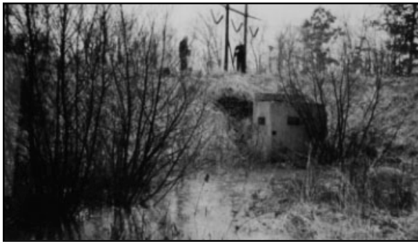
DESTABILIZING INFLUENCE. Trees on embankments and bottom areas will destabilize the BMP.
